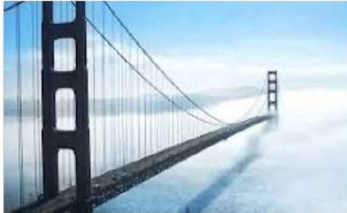
Bridge Seasonal-Decadal. Forecasts up to 24-36 months
